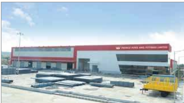
JOBNER - RAJASTHAN PIPES & WATER TANKS
